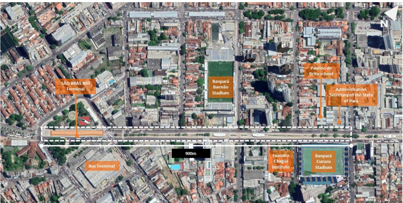
[b] Satellite view of the pilot location, including major buildings and services
